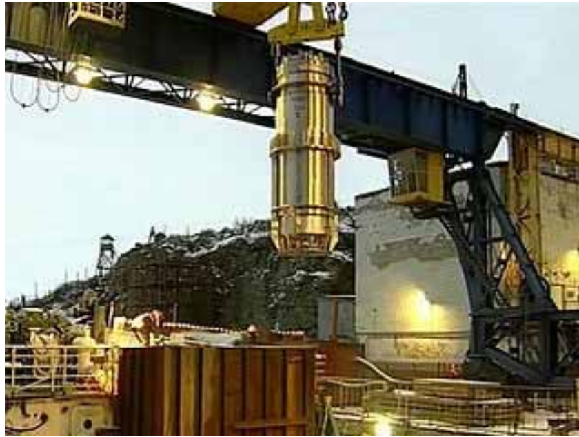
FIG. 3. Removal of submarine spent nuclear fuel from the former naval base at Gremikha for reprocessing at the Mayak plant in the Russian Federation.
