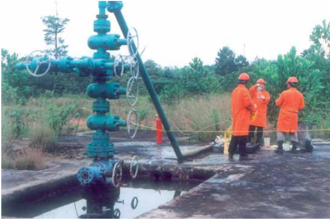
FIG. 1. Injection of tritiated water (HTO) as a tracer for interwell study at an oilfield in Indonesia.
