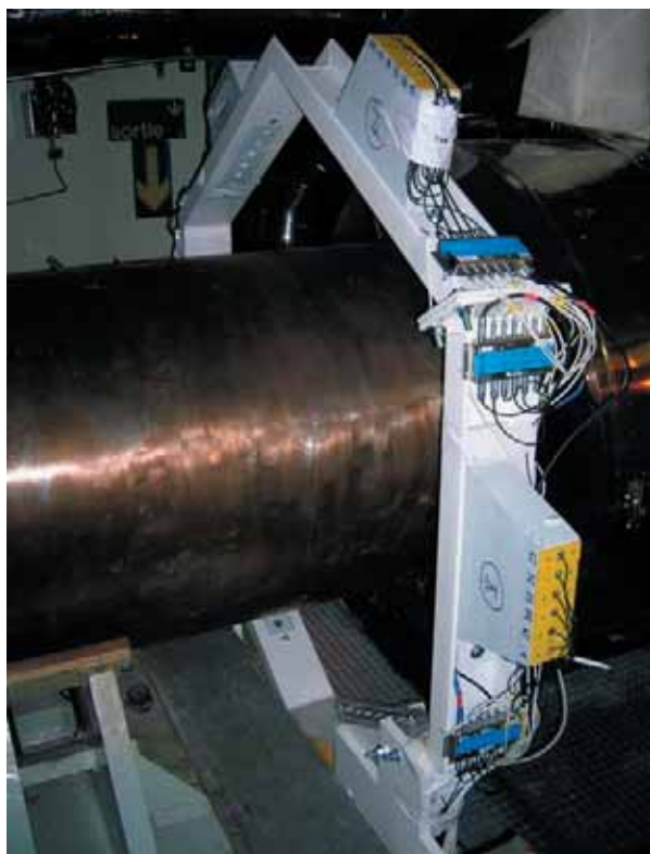
FIG. 2. A single photon emission computed tomography system in a French nuclear power plant. The system, installed around the primary circuit of a PWR, improves the estimation of nuclear thermal power in correlation with nitrogen-16 activity produced from oxygen-16 in water.
