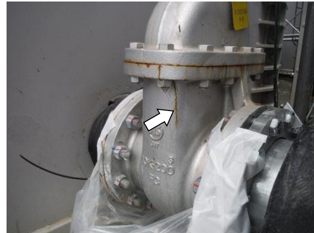
location of the crack
