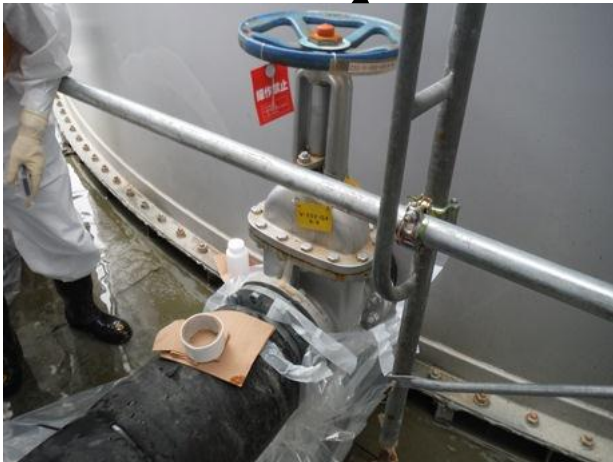
the valve where the leakage was found
