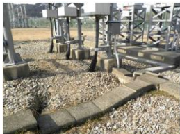
Okuma line 3L, Ground wire (disconnected)
