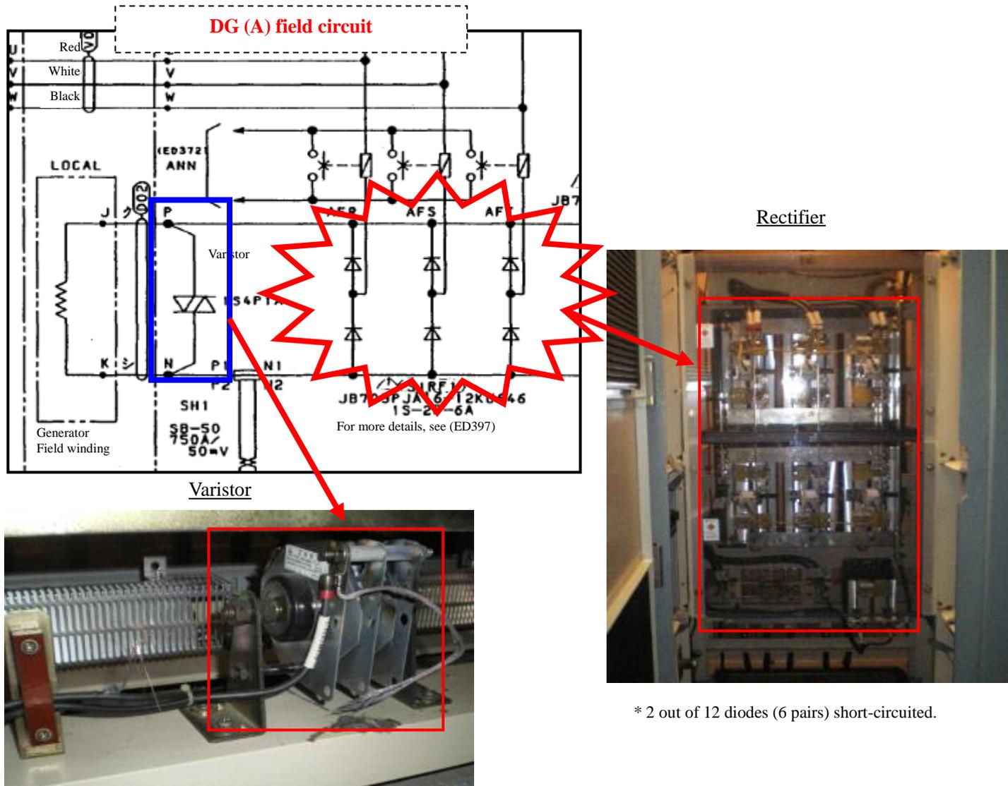
Fig. II-2-151 Onagawa Nuclear Power Station Unit 1 Damage to the DG (A) field circuit components
