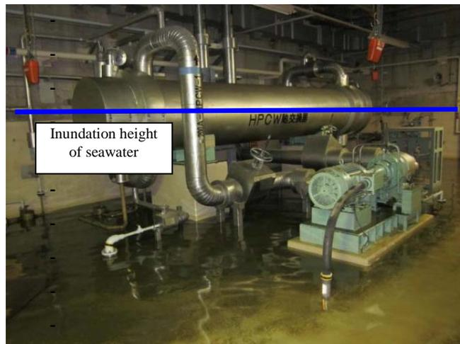
Seawater flooding in the HPCW heat exchanger chamber
