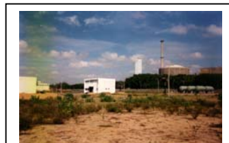
A 6300m 3 /d desalination plant is being connected to existing PHWR units at Kalpakkam, India. The desalination plant is a hybrid comprising of a reverse osmosis system and a multi-stage flash system.
