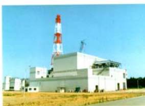
JAERI's HTTR has the capability to operate at a core outlet temperature of 950°C and is utilized to investigate technologies for advanced HTGRs, to demonstrate nuclear process heat applications, and to serve as an irradiation test facility for high temperature research activities. (Credit: JAERI)
