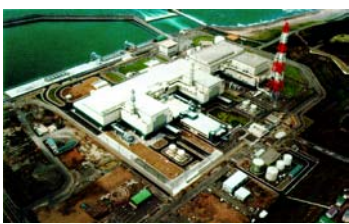
Tokyo Electric Power Company's Kashiwazaki-Kariwa Units 6&7 Two Advanced BWRs, which started commercial operation in November 1996 and July 1997 respectively. These plants were constructed by an international joint venture consisting of General Electric Nuclear Energy (USA), and Hitachi, Ltd, and Toshiba Corporation (Japan). (Credit: TEPCO)
