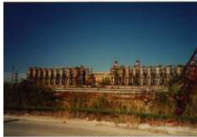
Evaporators at Aktau, Kazakhstan
