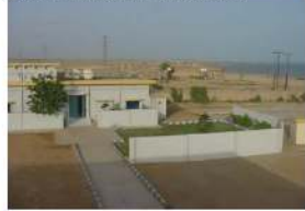
SWRO Plant at KANUPP, Pakistan
