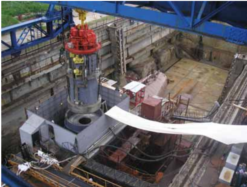
FIG. 6. The defuelling of a damaged nuclear submarine involved removal of the reactor core with liquid metal cooling.
