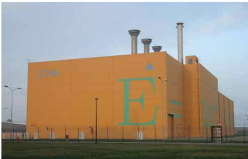
FIG. 1. A building for the interim storage of high level radioactive waste and spent fuel at the COVRA site, the Netherlands, which is designed to provide safe storage for at least 100 years.
