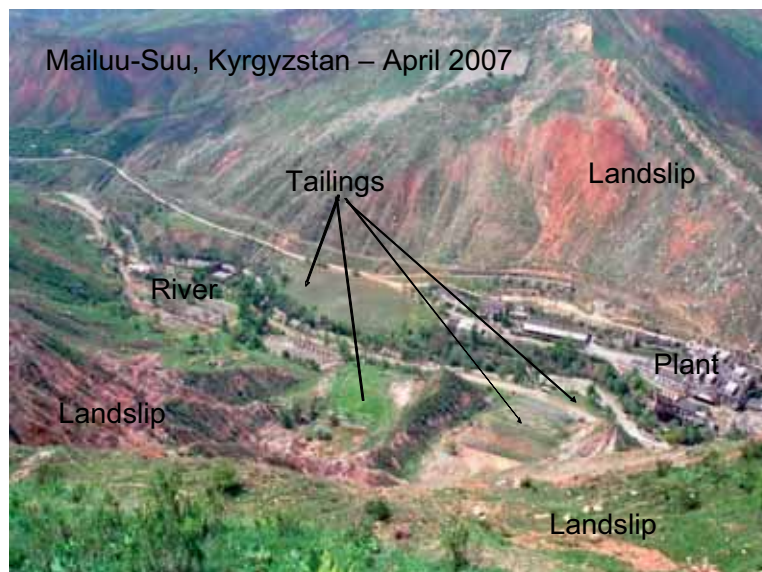
FIG. 5. The Mailuu-Suu site in Kyrgyzstan. The tailings piles are in the centre of the photograph and the potential landslips are on the left (red soil) and across the river on the hillside.
