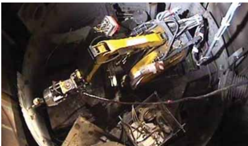
FIG. 3. Remotely operated liner removal at the SILOE research reactor in Grenoble, France.
