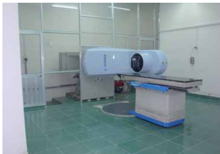
FIG. 5. The Bhabhatron radiotherapy unit donated by India as installed in a local hospital in Can Tho Province, Vietnam.
