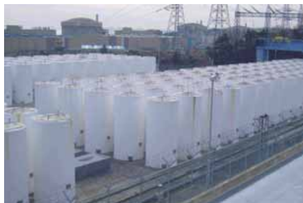
FIG. 2. Dry storage casks at the Wolsong nuclear power plant site in the Republic of Korea.
