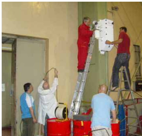
FIG. 2. Installation of remote monitoring equipment to improve the physical protection of a nuclear facility.
