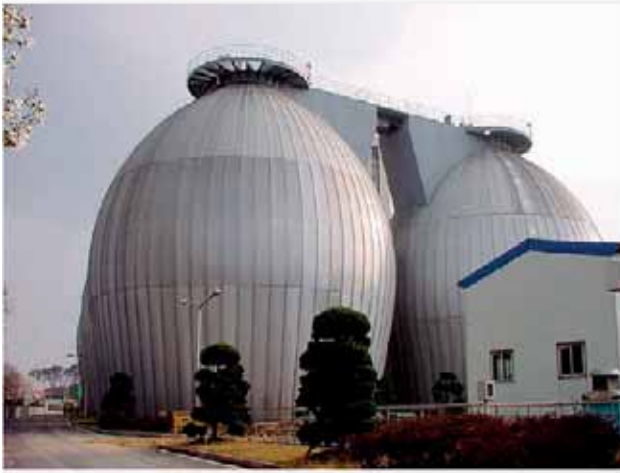
FIG. 1. Investigation of sludge digesters in a wastewater treatment plant in the Republic of Korea using scandium-46 as a tracer.
