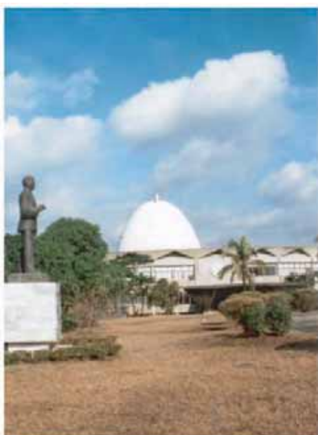
FIG. 1. The Philippine research reactor PRR-1, which will be used as a model for the Research Reactor Decommissioning Demonstration Project.
