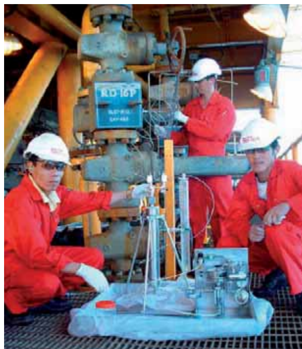
FIG. 1. Radiotracer injection at an offshore oil platform in Vietnam.
