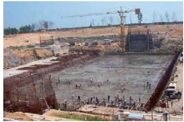
FIG. 2. Construction work on the fast breeder reactor at Kalpakkam, in India.
