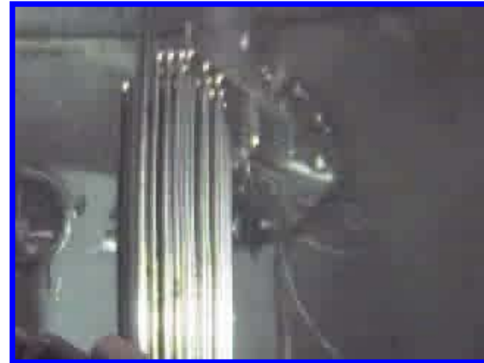
PRHR Heat Exchanger
