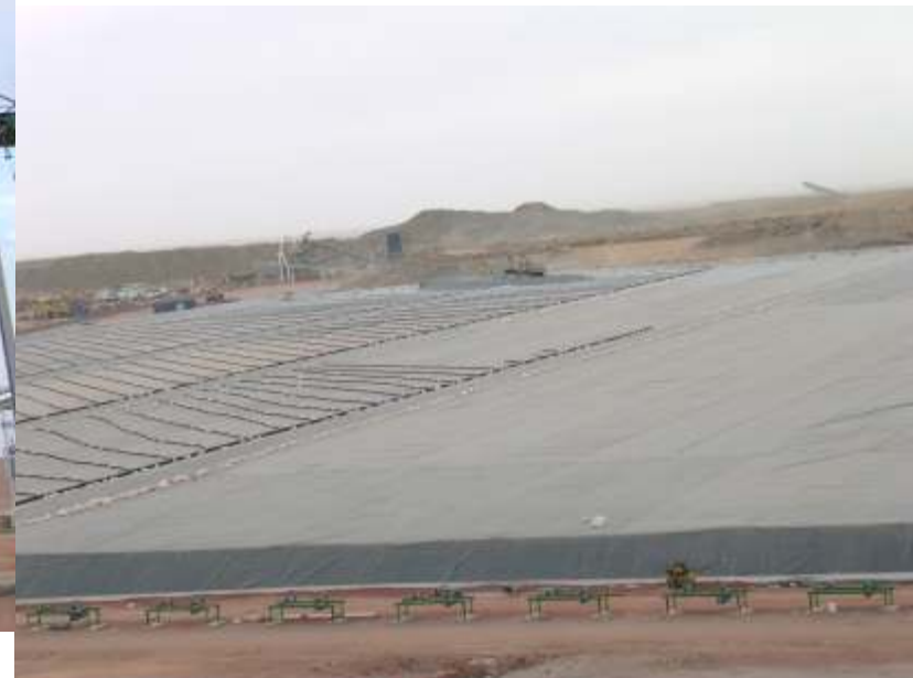
1 st Pad construction (176500 m 2 )
