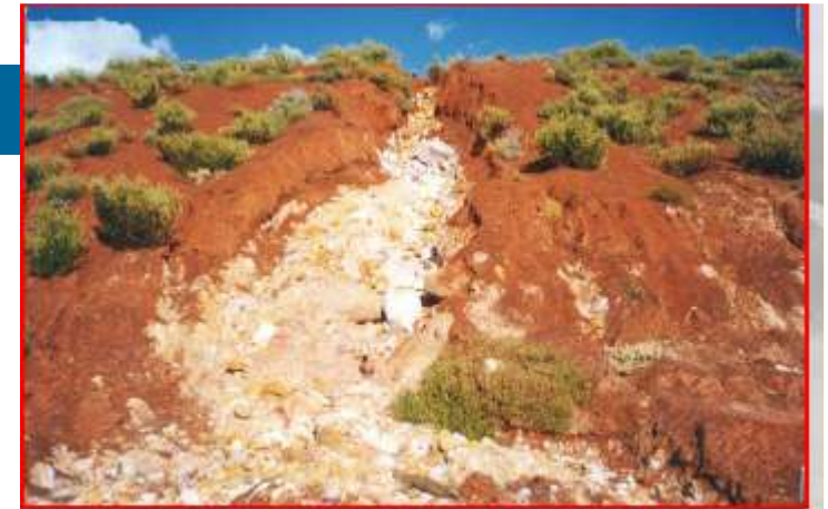
Erosion due to poorly designed water-control structures
