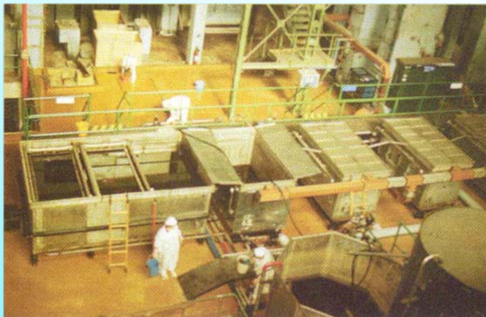
High-capacity decontamination facility
