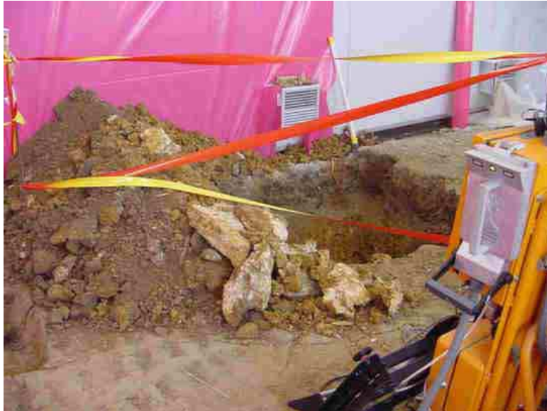
Cleanup operations inside MOCA
