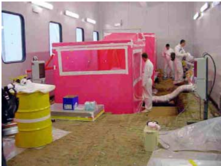
Cleanup operations inside MOCA
