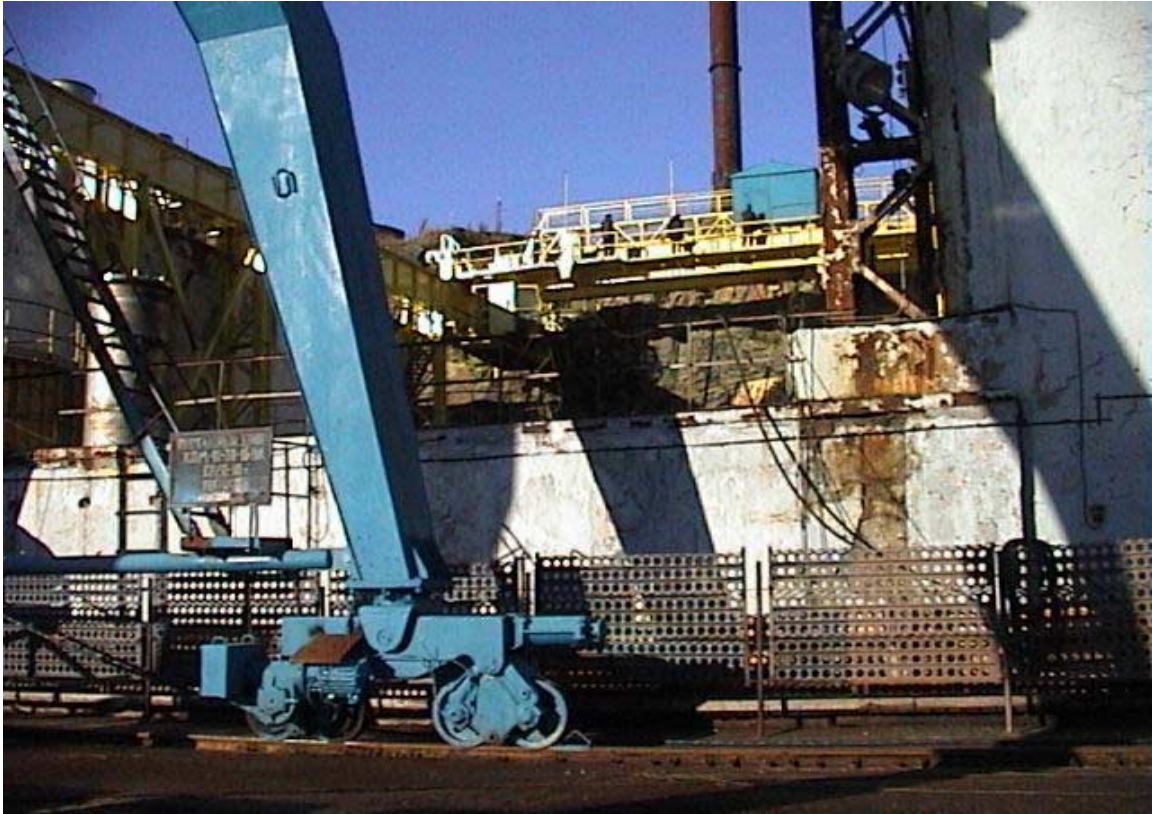
Photo 4. The MK 20/5 bridge crane
