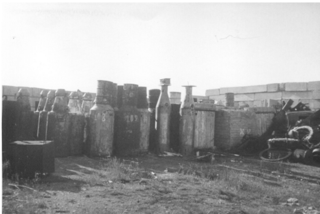
Fig. 3. SRW storage pad
