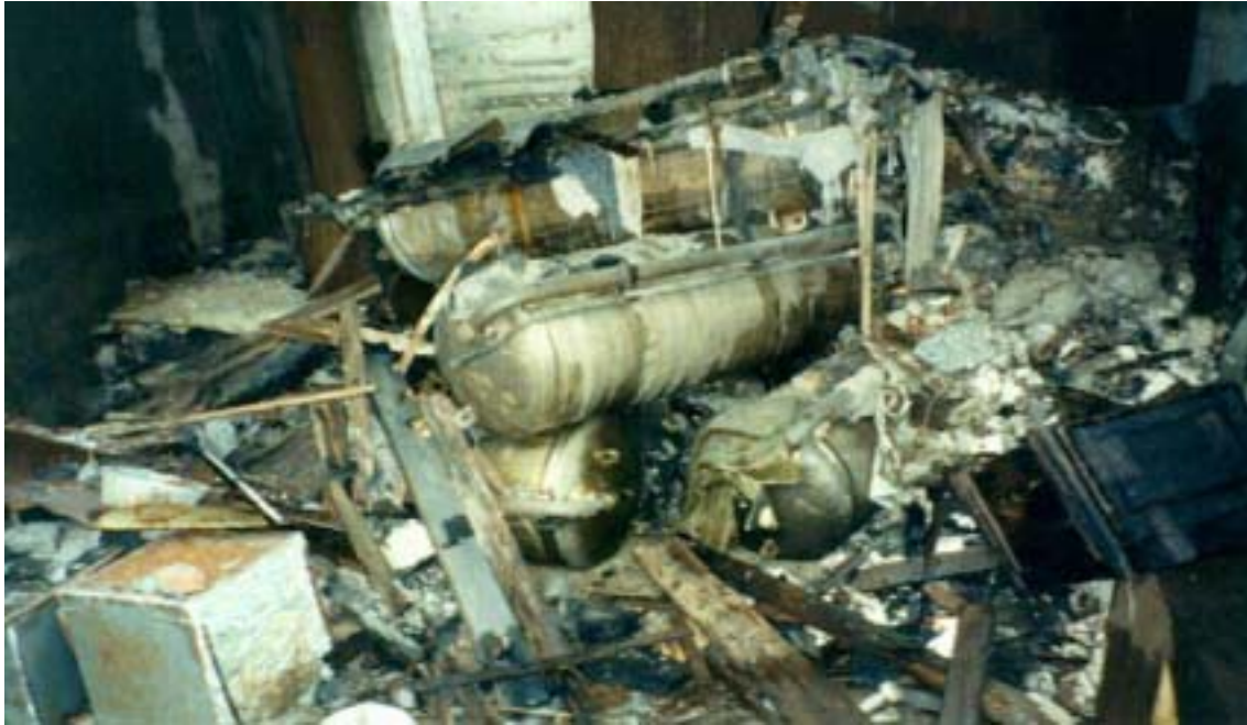
Fig. 6. View inside cell #1
