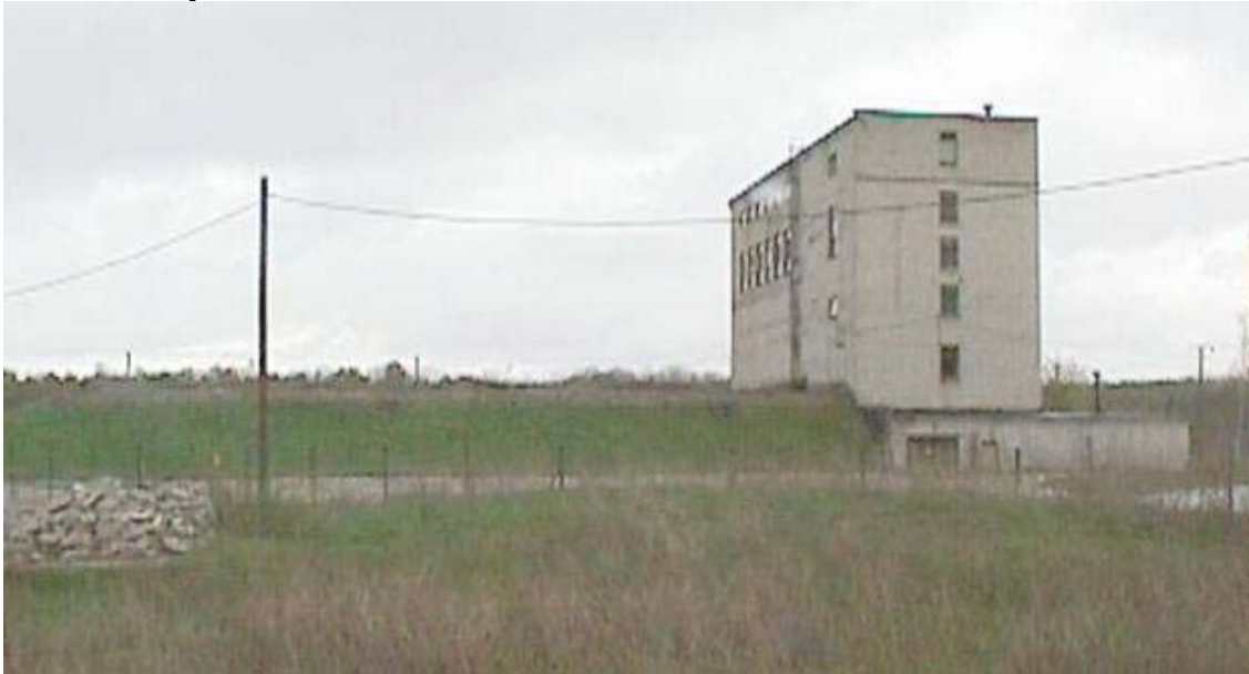
Fig. 39. Building 303, Liquid Waste Treatment Building, and Tank farm
