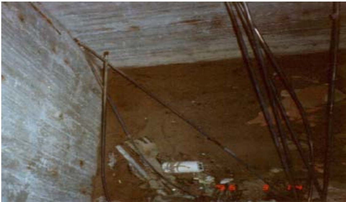
Fig. 8. Control rods and sources in cell #5
