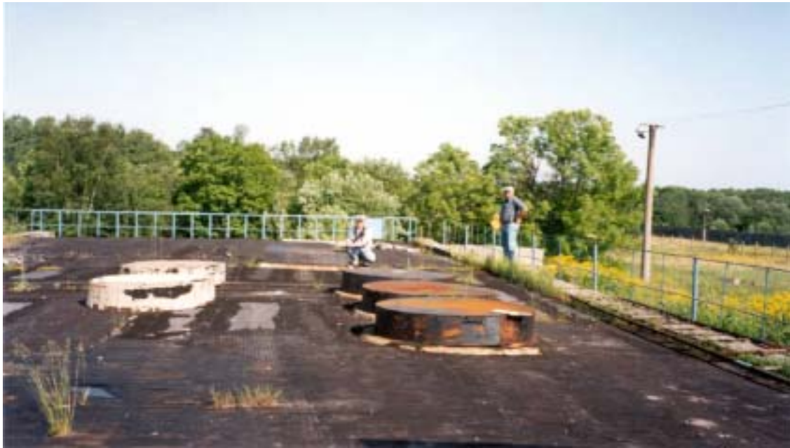
Fig.3. The roof of SWS
