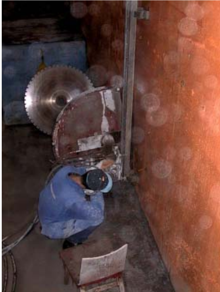
Fig. 17 The concrete saw, mounted vertical, cutting an opening through a wall.
