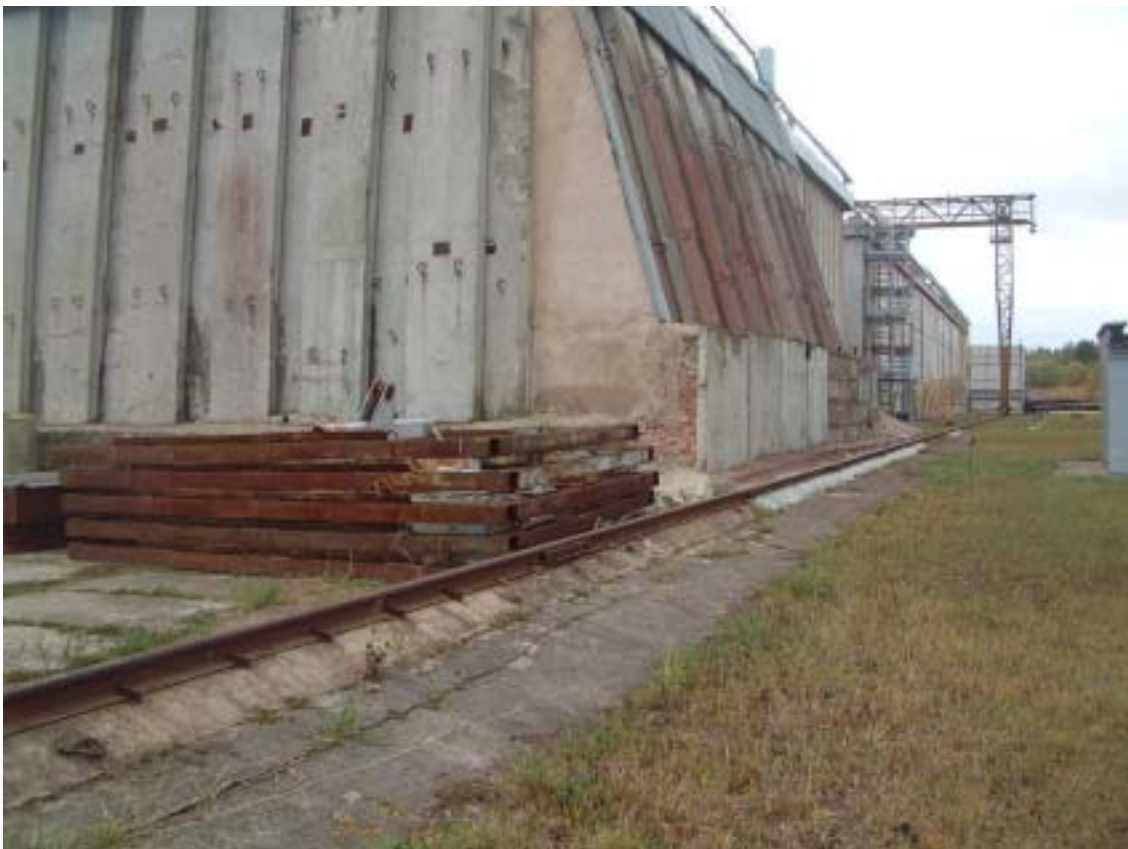
Fig. 51. Strengthening of building 157 SE corner
