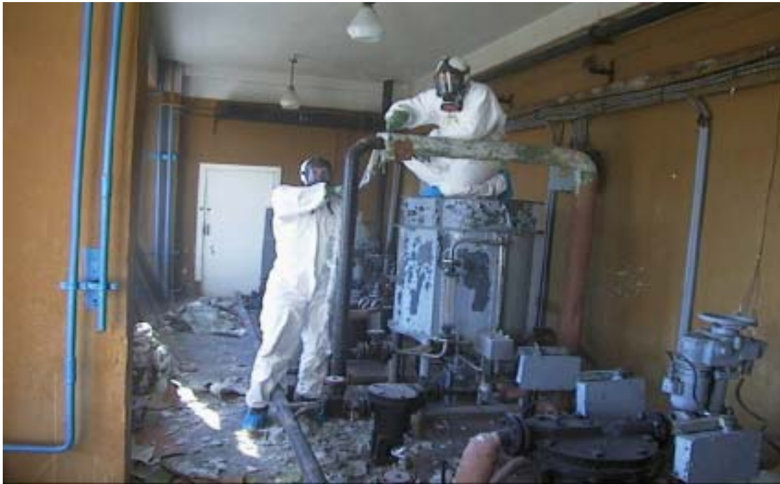
Fig. 41. Removal of asbestos
