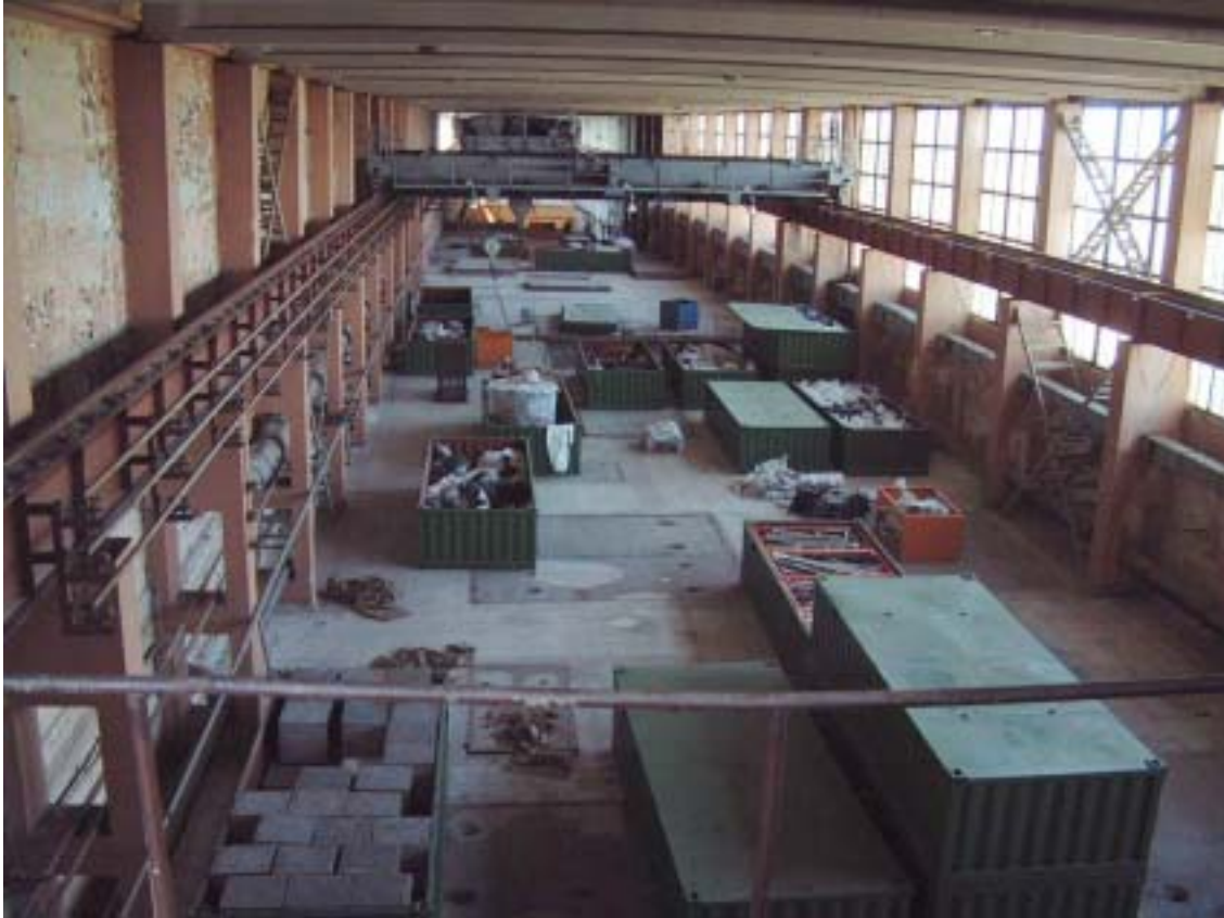
Fig. 48. Temporary container storage
