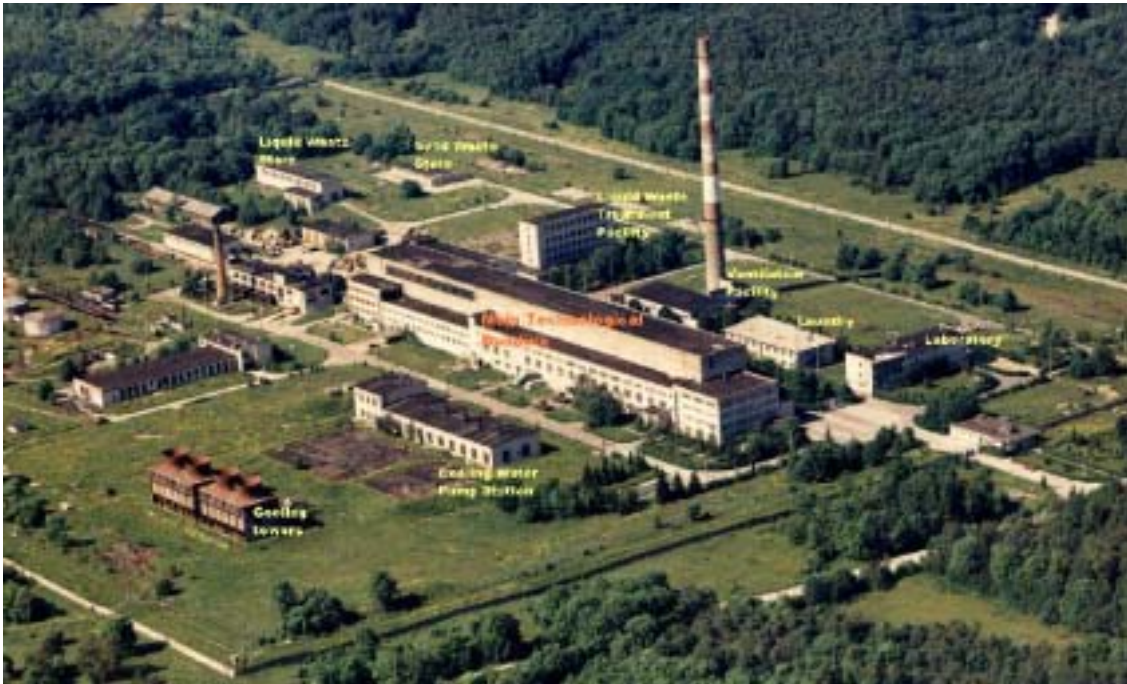
Fig.2. Aerial view of the Paldiski site in year 1995
