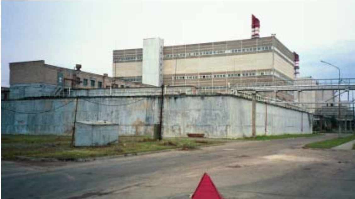
Fig. 52. Storage for bituminised waste
