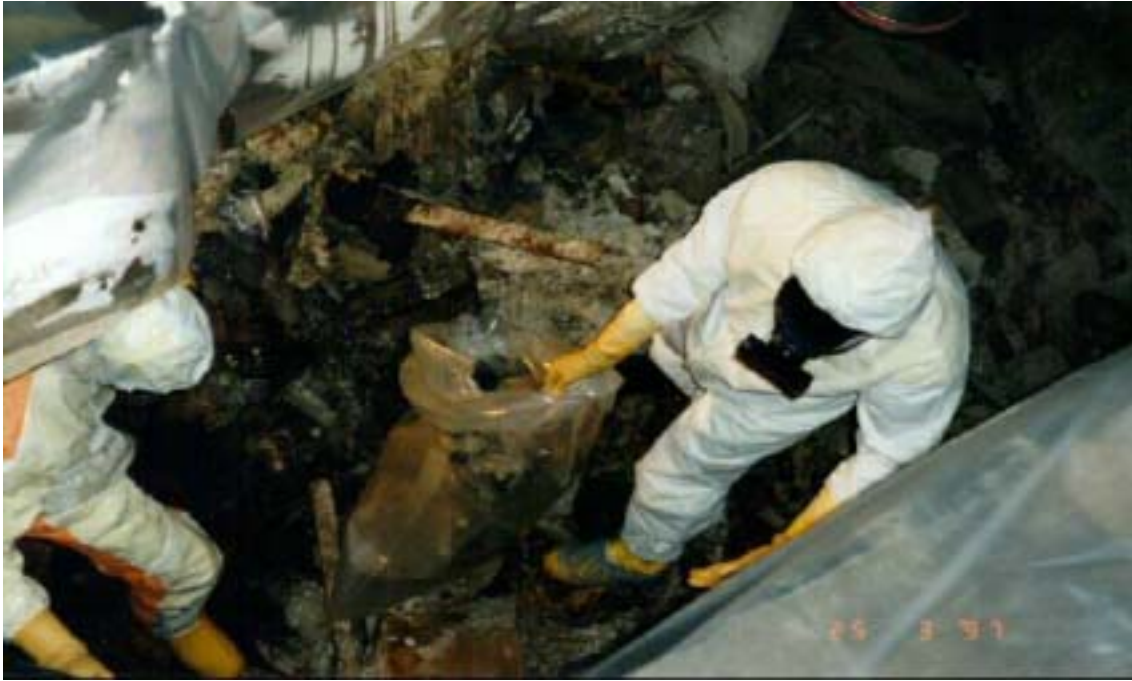
Fig. 14. Manual work in cell #4A
