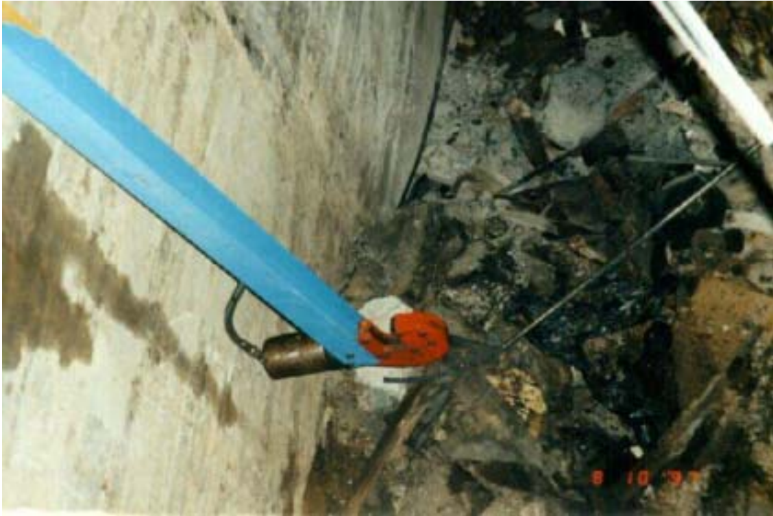
Fig. 27. The hydraulic shear in cell #1
