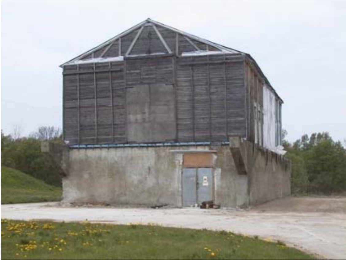
Fig. 16. The opening in the ground wall
