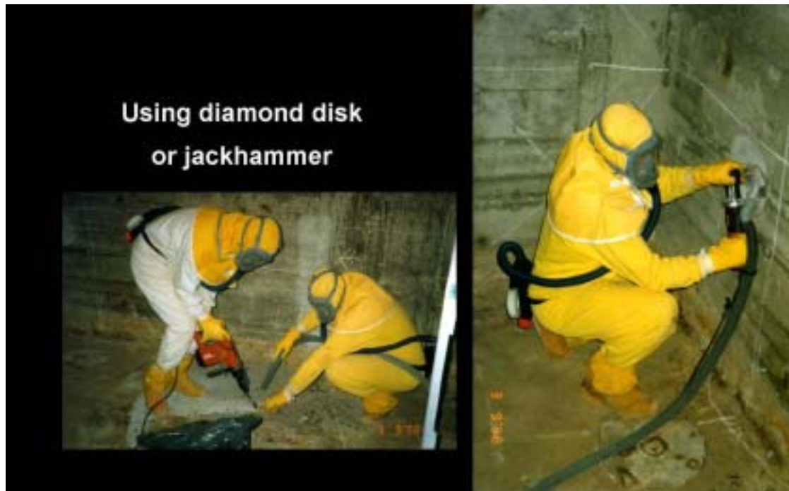
Fig. 42. Concrete decontamination work
