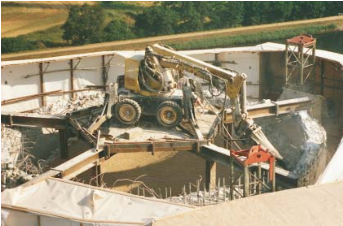
Fig. 47. A BROKK demolition robot
