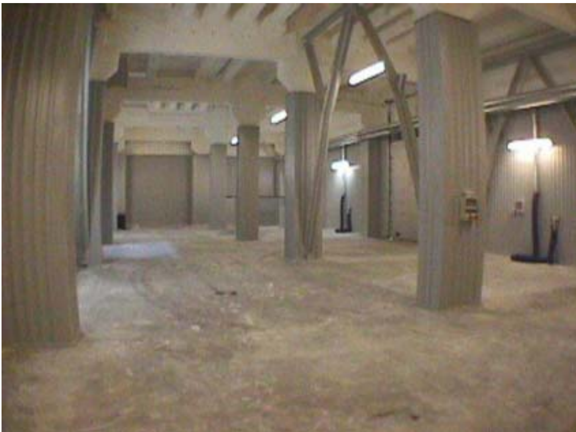
Fig. 38. Waste handling area in the annex building
