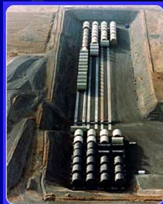
Fluor constructed – Nuclear Navy Reactor storage
