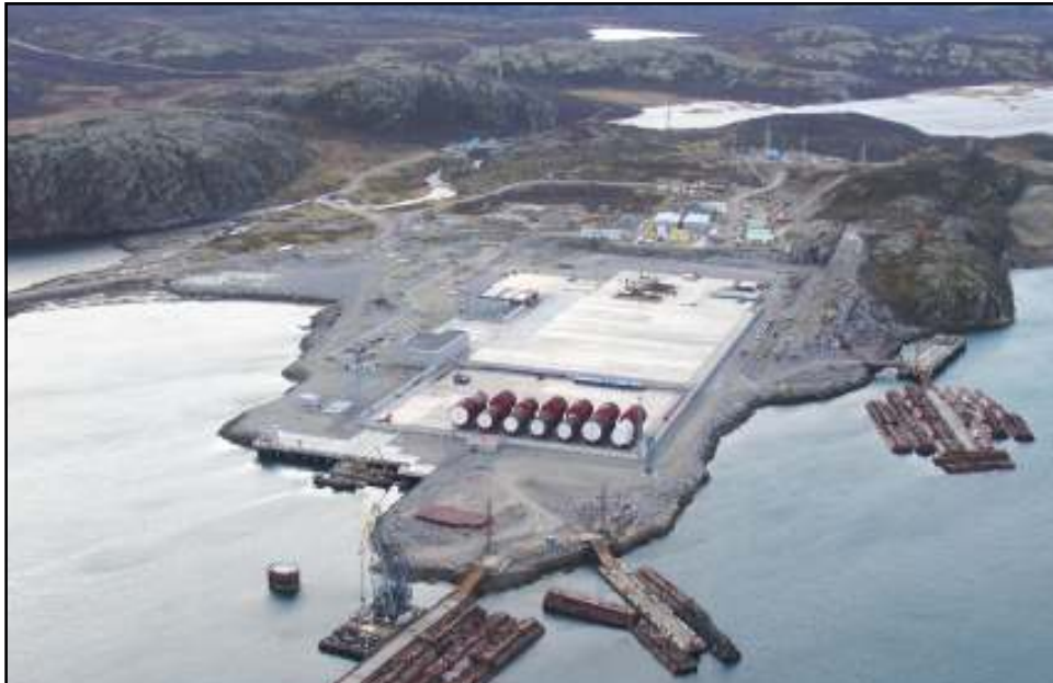
General view of the radioactive waste management complex
