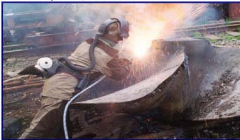
Fig. 4. Gas cutting during submarine dismantling
