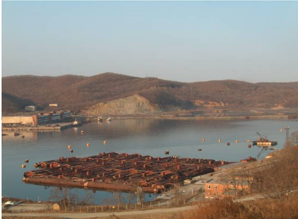
Figure 5. Storage of the reactor compartments afloat in the Razboynik Bay
