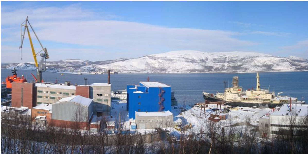
Figure 4. Storage facility for unprocessable SNF at the Atomflot site in Murmansk
