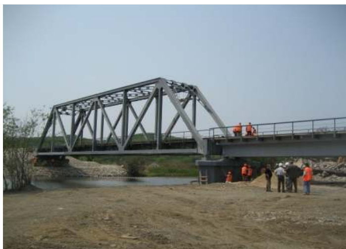
A Canadian funded bridge completed in May 2009 as a part for the railway line for SNF transportation from the Far-East
