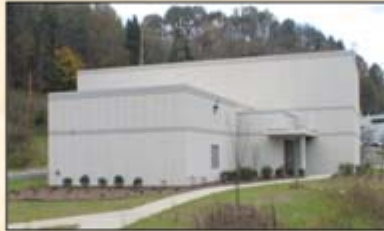
High-resolution approach: fully automated remote operation in room isolated from vibration, EM fields, \Delta T and people
