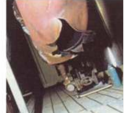
Main feedwater piping rupture at Loviisa-1, VVER, 465 MWe, 1990
