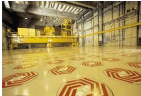
Figure 4. The storage hall for vitrified waste at La Hague.
