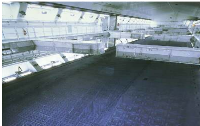
Figure 1. The pool at the CLAB wet storage facility in Sweden.
