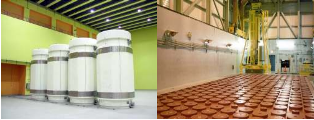
Figure 2. Dry fuel storage technologies: casks at the ZWILAG facility in Switzerland (left) and the Fort St. Vrain vault in the USA (right).
